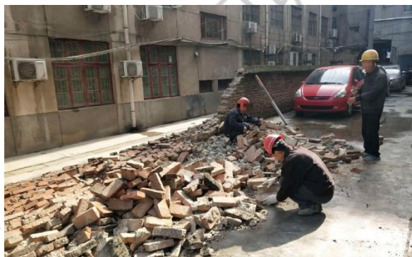
3D-1-4-1 拆除原有围墙
