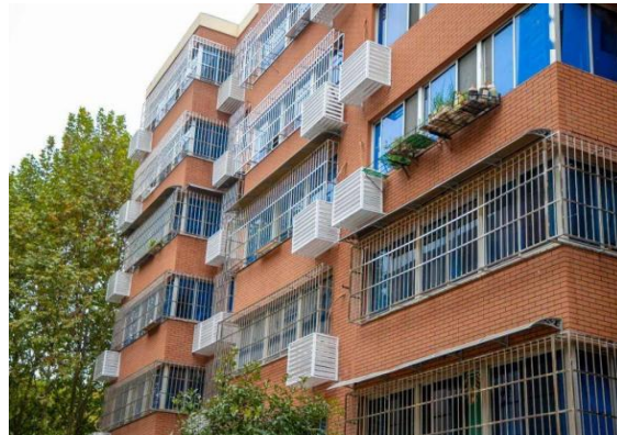
1D-3-1-3 空调机架更换
